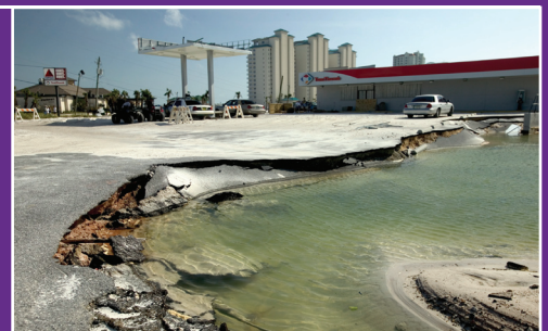
Navarre Beach, FL: Damage to homes, businesses and infrastructure due to Hurricane Dennis. FEMA photo/Andrea Booher
