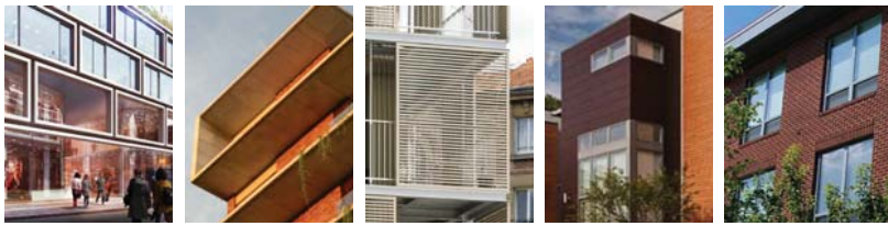
CONCRETE BRISE SOLEIL CONCRETE EYEBROWS & FINS ALUMINUM GARAGE SCREEN SCORED STUCCO FINISH ALUMINUM WINDOWS
