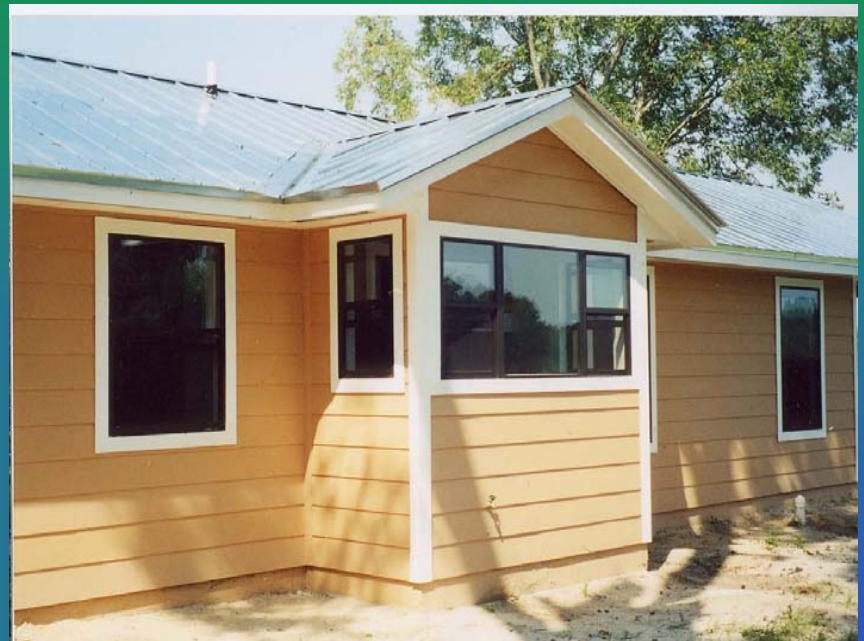
Aachua County Housing Authority Green House
